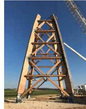
Hybrid masts wood/steel
