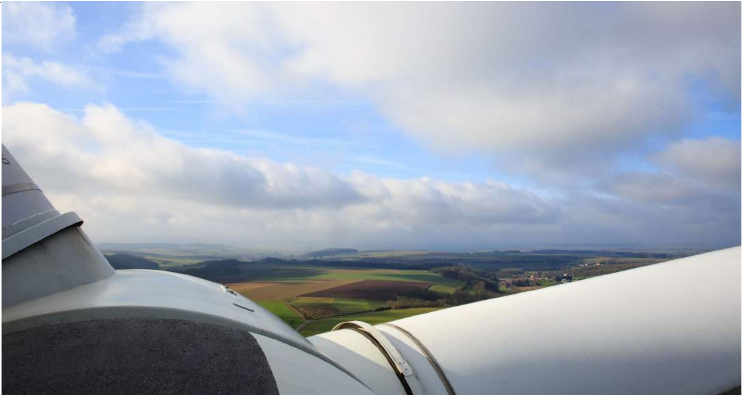
Fiefs wind farm in France
